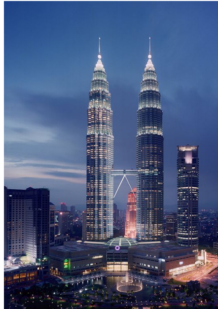
Fig. 7 – Petronas Towers (fonte: https://www.wsp.com/en-SG/projects/petronas-towers-and-kuala-lumpur-city-centre )
