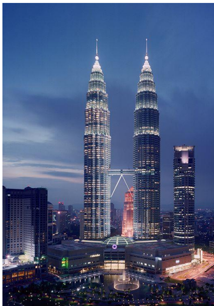
Fig. 7 – Petronas Towers (fonte: https://www.wsp.com/en-SG/projects/petronas-towers-and-kuala-lumpur-city-centre )
